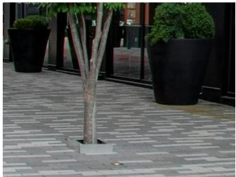
Description: Paver-Grate Pavement Suspension System with Integrated Tray System Paver Grate System by Ironsmith, <u>www.ironsmith.cc</u>
