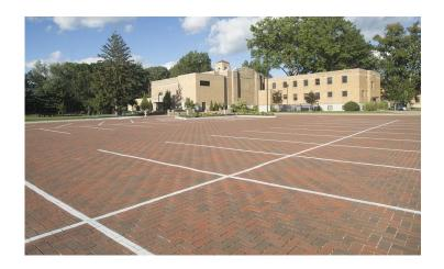
Description: Clay brick paver with chamfered edges and spacer lugs, 4"x8"x2-3/4", Red blend City Line Series Pavers by Belden Brick Company, <u>www.beldenbrick.com</u>
